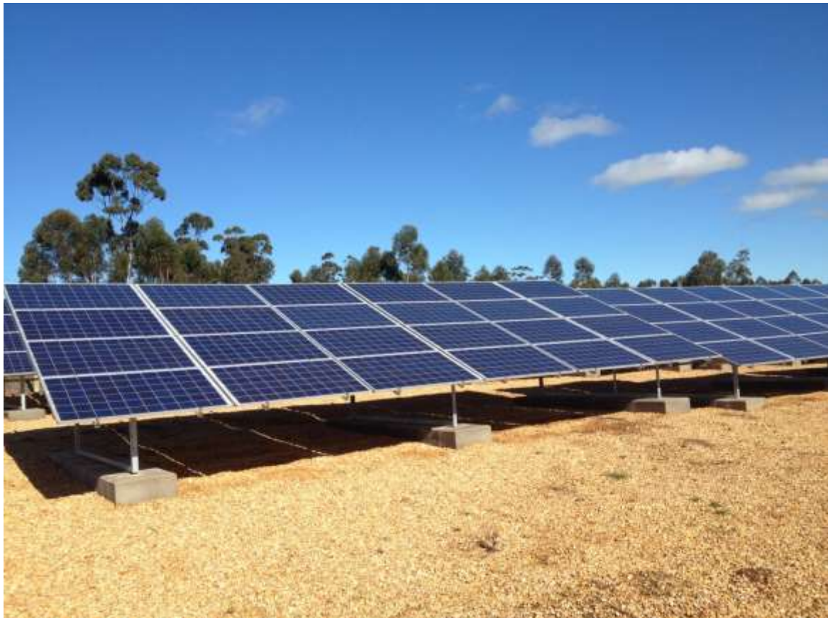
Figure 9-2: Riversdale's 33 kWp PV system.
